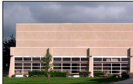
The roof of the gym indicates an attempt to use standard campus architectural vocabulary on a large flat roof structure. Window and column forms recall those used on classroom buildings.
