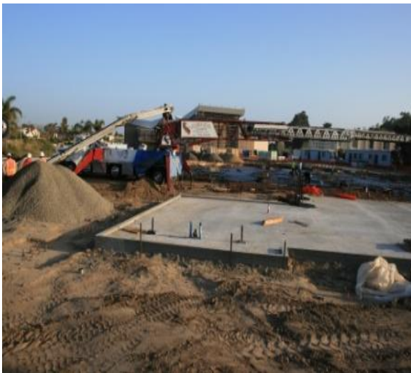
Concrete slab @ west wing
