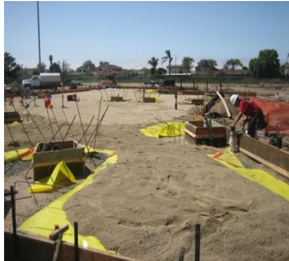
Concrete slab preparation
