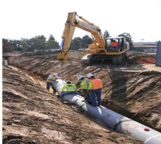
Storm Drain work
