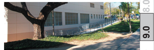
View of a ramping system on the eastside of the gym which is an example of accessible circulation (above).
