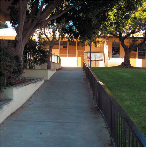
View of ramp along the Art's Courtyard (above).
