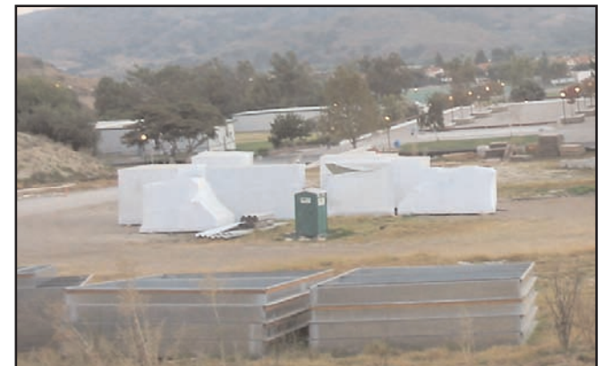
L/LR construction staging area
