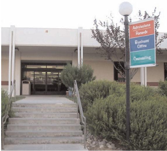
Building Administration west entrance with banners
