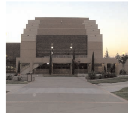
Theater colonnade constructed using colored and textured concrete masonry block.
