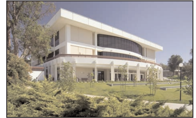
L/LR South facade
