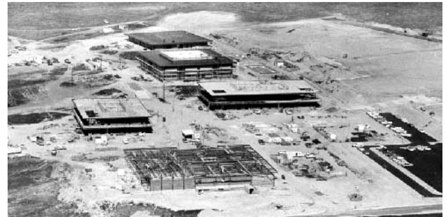
Construction photograph showing the Student Center, the Technology building, the Physical Science building, the Library and the Administration building under construction.
