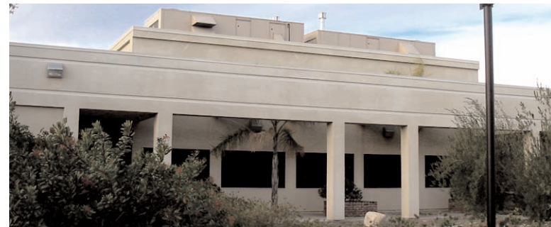
Communications Building exterior east facade with stucco mechanical screen
