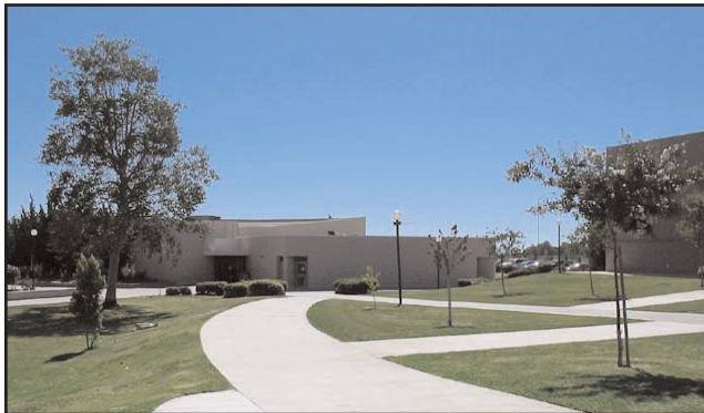
Northeast corner entrance to the Music building
