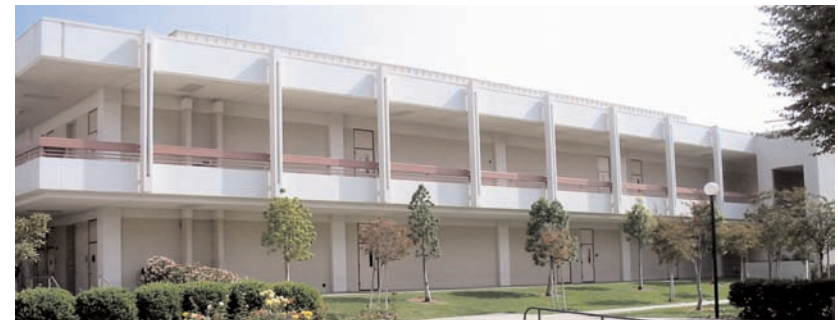
Top Left: LMC Building second floor railing and pre-cast concrete fin. Top Right: Student Center south exterior colonnade. Bottom: LMC south facade with colonnade
