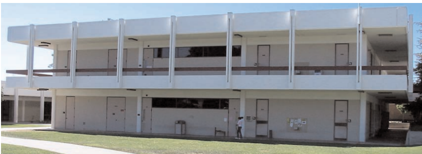
Existing Technology Building pre-cast panel design at the eaves
