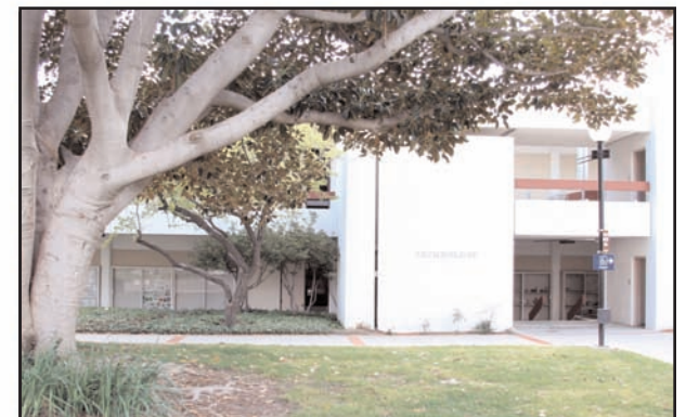
Courtyard by Technology building
