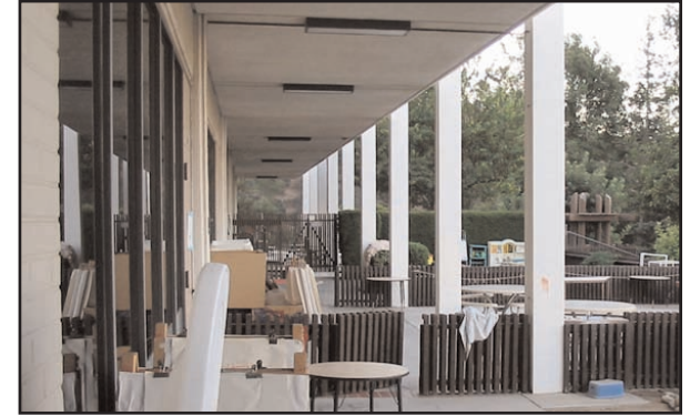
Existing CDC children's playground
