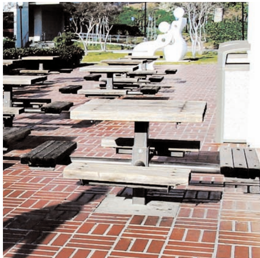
Floor mounted wood bench and table.
