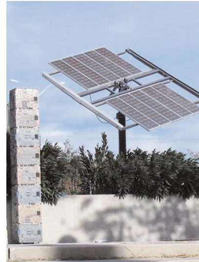
Photovoltaic installation at north campus entrance
