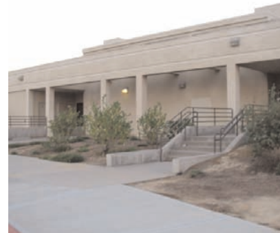
Wood framed and stucco finish colonnade at the Communications building
