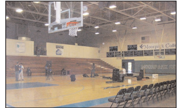
Gym interior - New Bleachers being installed
