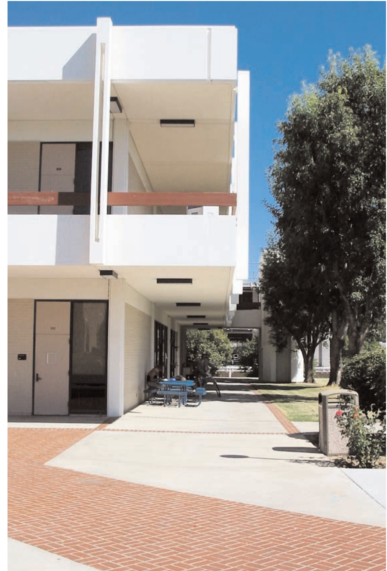
Building HSS Exterior Walkway. 1975 two-story instructional building.
