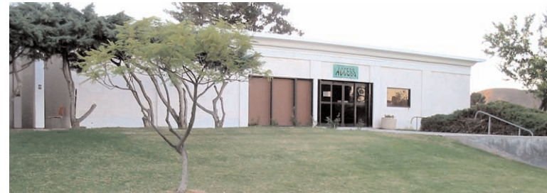
ACCESS Center exterior west facade
