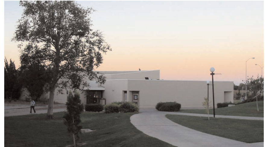
The Music Building is the only building on campus with a different geometry and sloped rooflines. The building was completed in 1975.
