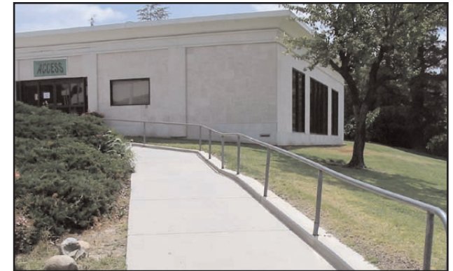
Various ramps and pedestrian accesses need to meet accessibility codes
