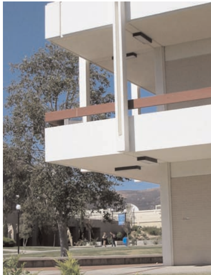
Covered walkway at the second floor of the Humanities Building
