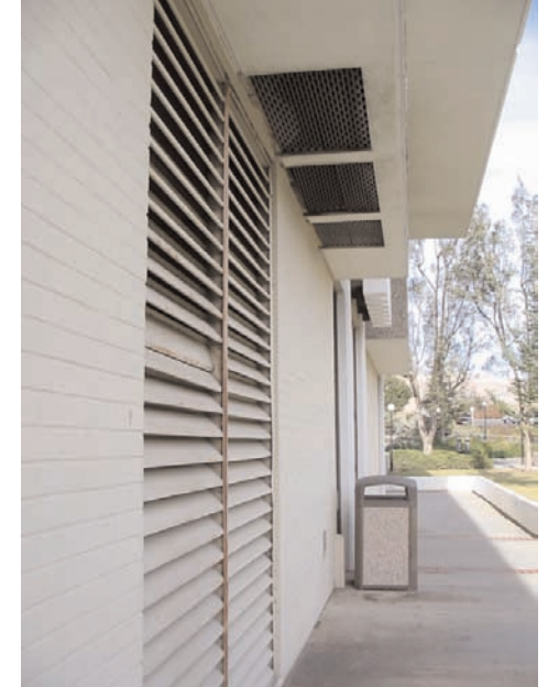
Former Library building mechanical room exterior vents at north facade
