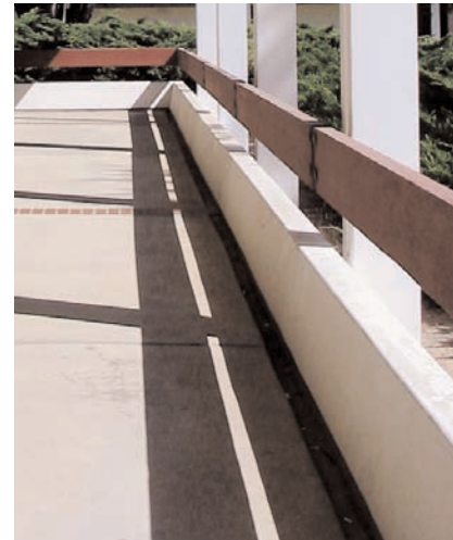
Original wood guardrail and pre-cast detail at the first floor Administration building
