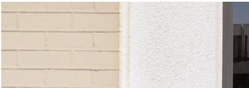
Administration Building exterior painted brick finish, concrete clad and stucco column finish, and store-front window finish at facades.
