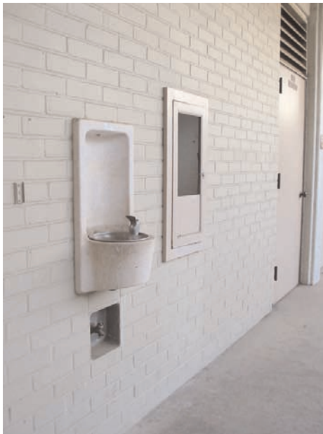
Built-in water fountain and recessed water hose connection and fire extinguisher onto the side of the building at exterior corridors
