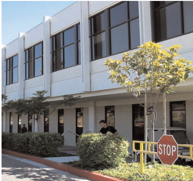
LMC Building north facade
