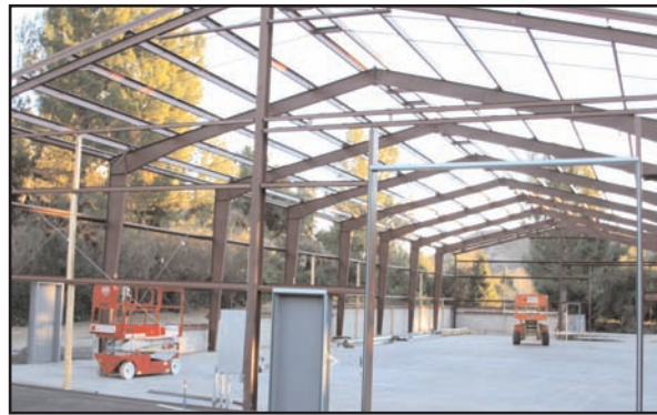
Warehouse under construction
