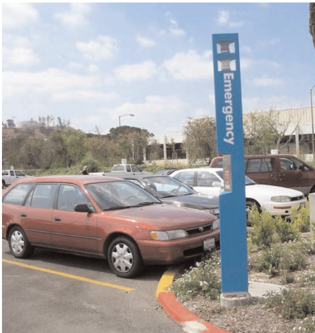
Existing emergency call station, parking lot B
