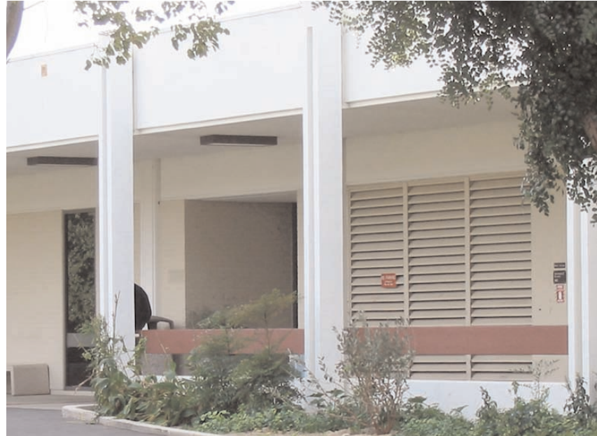
Administration building mechanical room exterior vents at north facade
