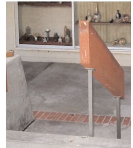
Original wood handrail
