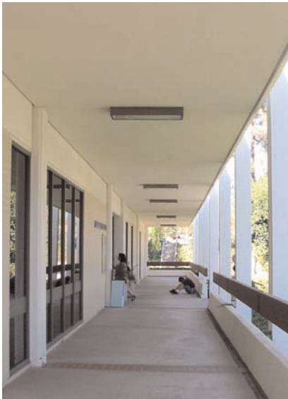
Covered walkway at the first floor of the Administration Building
