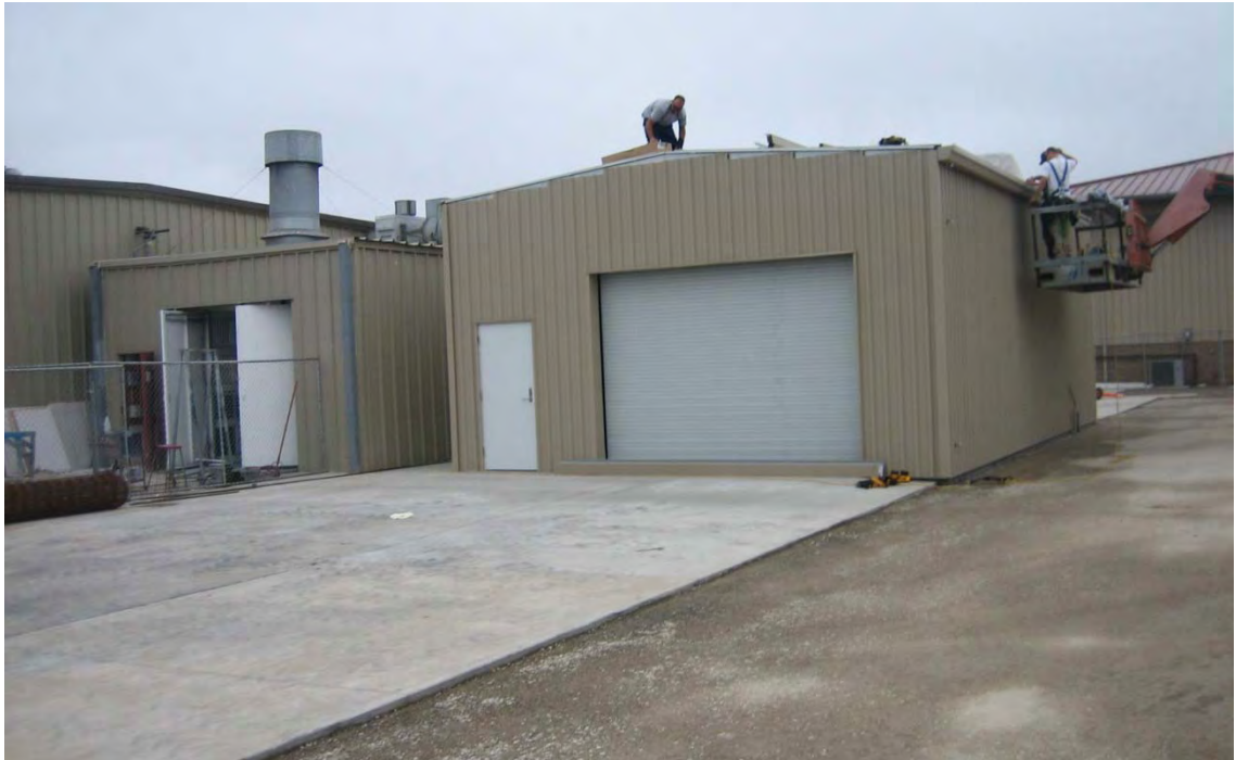
Auto Tech: New Metal Building Enclosure Around New Paint Booth
